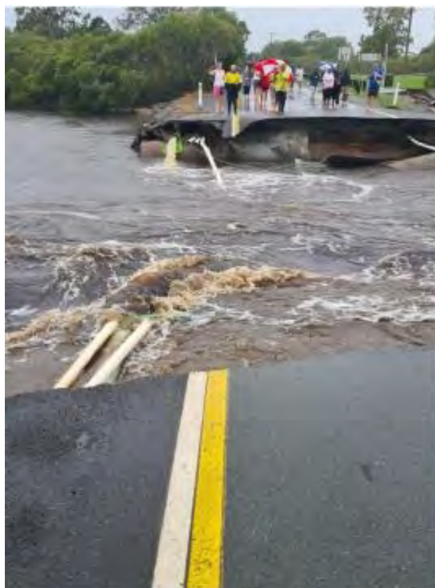
Photo 3-8: Damaged fire duct alongside a washed-out bridge, NSW/QLD Border region 470
