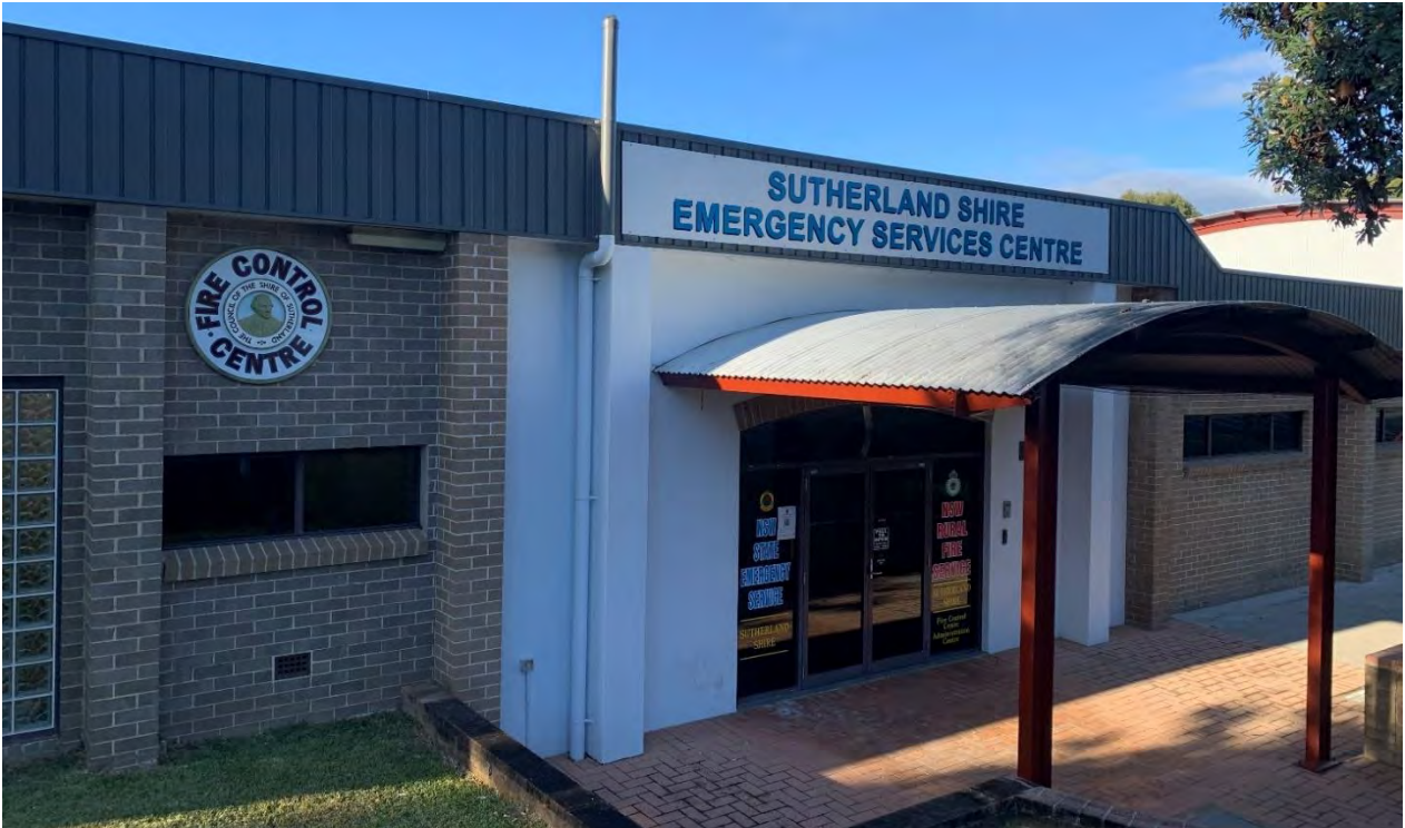
Photo 4-9: Sutherland Shire Emergency Service Centre. Source: Flood Inquiry Secretariat.
