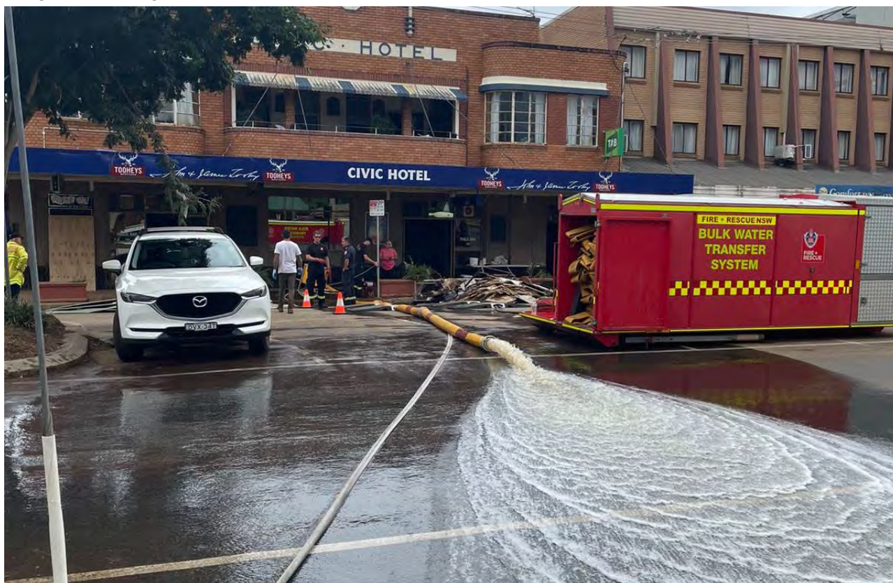
Photo 4-1: Hytrans high-capacity pump in Lismore.
