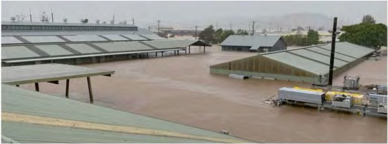
Photo 3-7: Essential Energy's Lismore depot on 28 February 2022.
