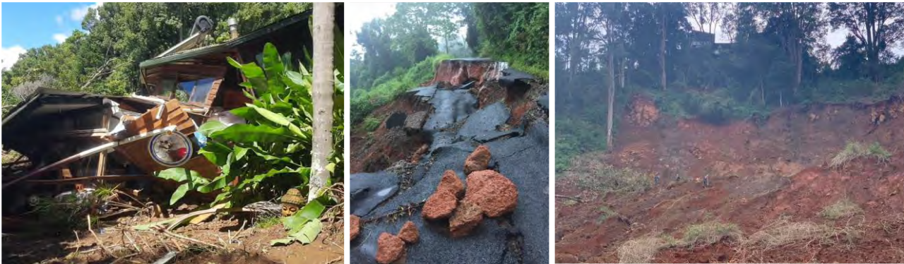
Photos 7-1: L-R: Collapsed home in Moondani; Damage to Tuntable Creek Road between Beardow Road and Rose Road; Landslip at Tuntable Coop. Source: Nimbin Community Response and Recovery Team.
